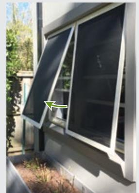
*Invisi-Scape easily opens outwards to allow for a quick escape in an emergency.*
